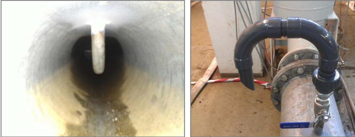
Figure 7 : Isokinetic sampling port “Pitot” type installations, left: inside main pipe with view upstream; right: sampling port with valve
